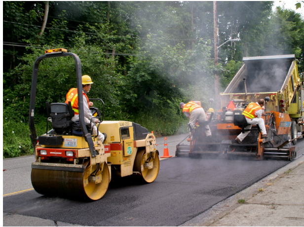
SR 7 Paving Project
